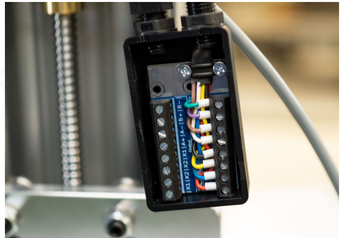
Fig. 5: Connected motor strands in the terminal box
