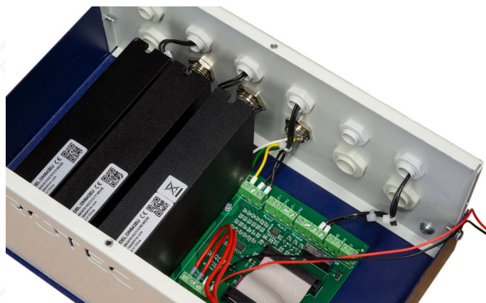
Image 17: Attached power amplifiers
