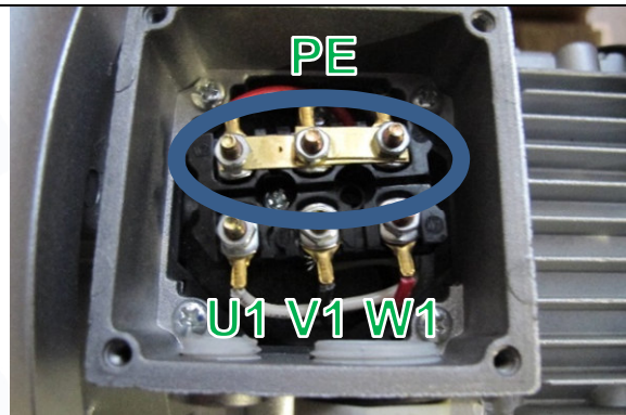
Fig. 2 Star bridge for 400 V operation
